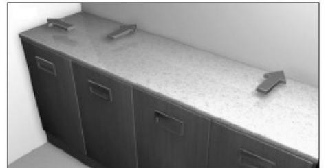
We suggest that an allowance of 10mm is made to accommodate a worktop overhang on an exposed worktop or show ends. Use a belt sander to remove the final material and to avoid saw chips. If necessary, hand finish the cut edge using a suitable grade of sandpaper.
