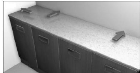
Position the worktop on the units and push it up against the wall to enable you to mark and measure for cutting. If the worktop is to be scribed to the wall, do so using a compass and pencil.
